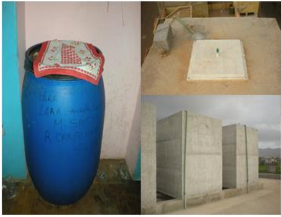
Figure 9: Domestic tanks used for storage of water
